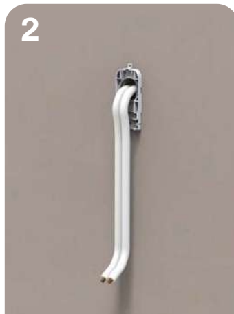
Insert the refrigeration lines and the power cable into the wall hole
