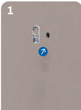
Fix the rear part of the aesthetic flange in correspondence with the wall hole
