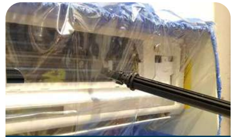
Battery cleaning through cleaning machine hole
