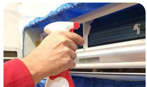
Battery cleaning without protective cover
