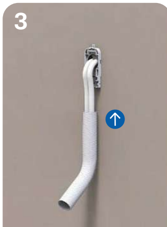
Place the refrigeration pipes and the power supply in the corrugated protection pipe
