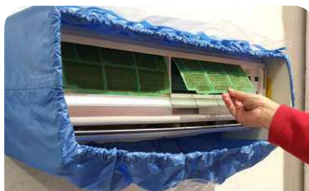
Removing the filters
